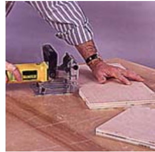
10--Use your worktable as a registration surface when cutting the slots in the storage box partition panels.
